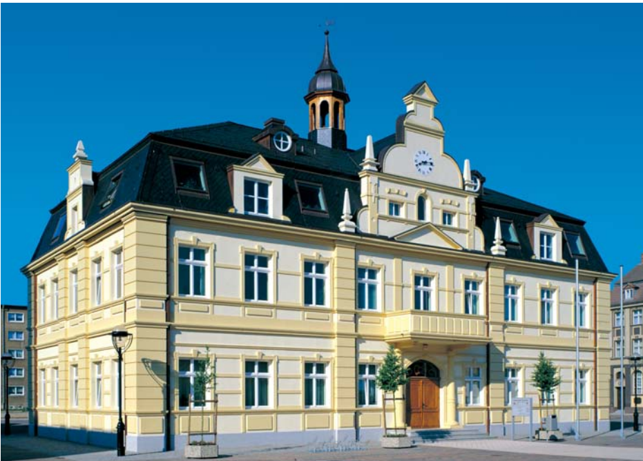
Town hall, Demmin Architectural firm: Bauplan Consult GmbH, D-Neubrandenburg
